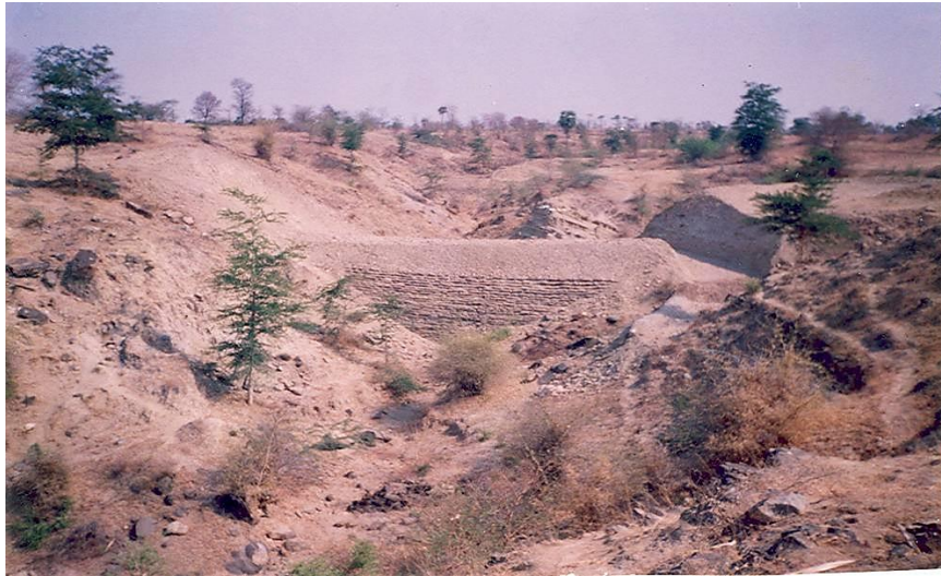
Sedimentary Storage dam (Front view )
