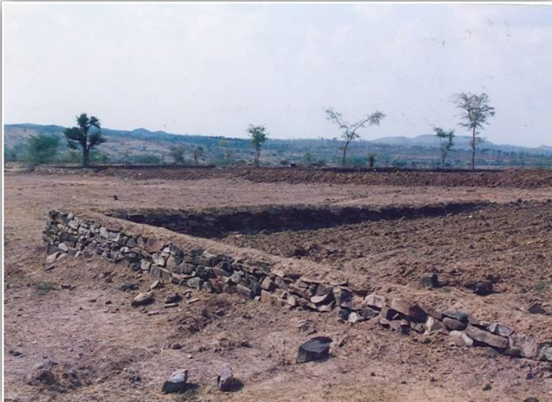
Traditional spillway with apron (drop structure) in Kenbarte - Kyaukpadaung
